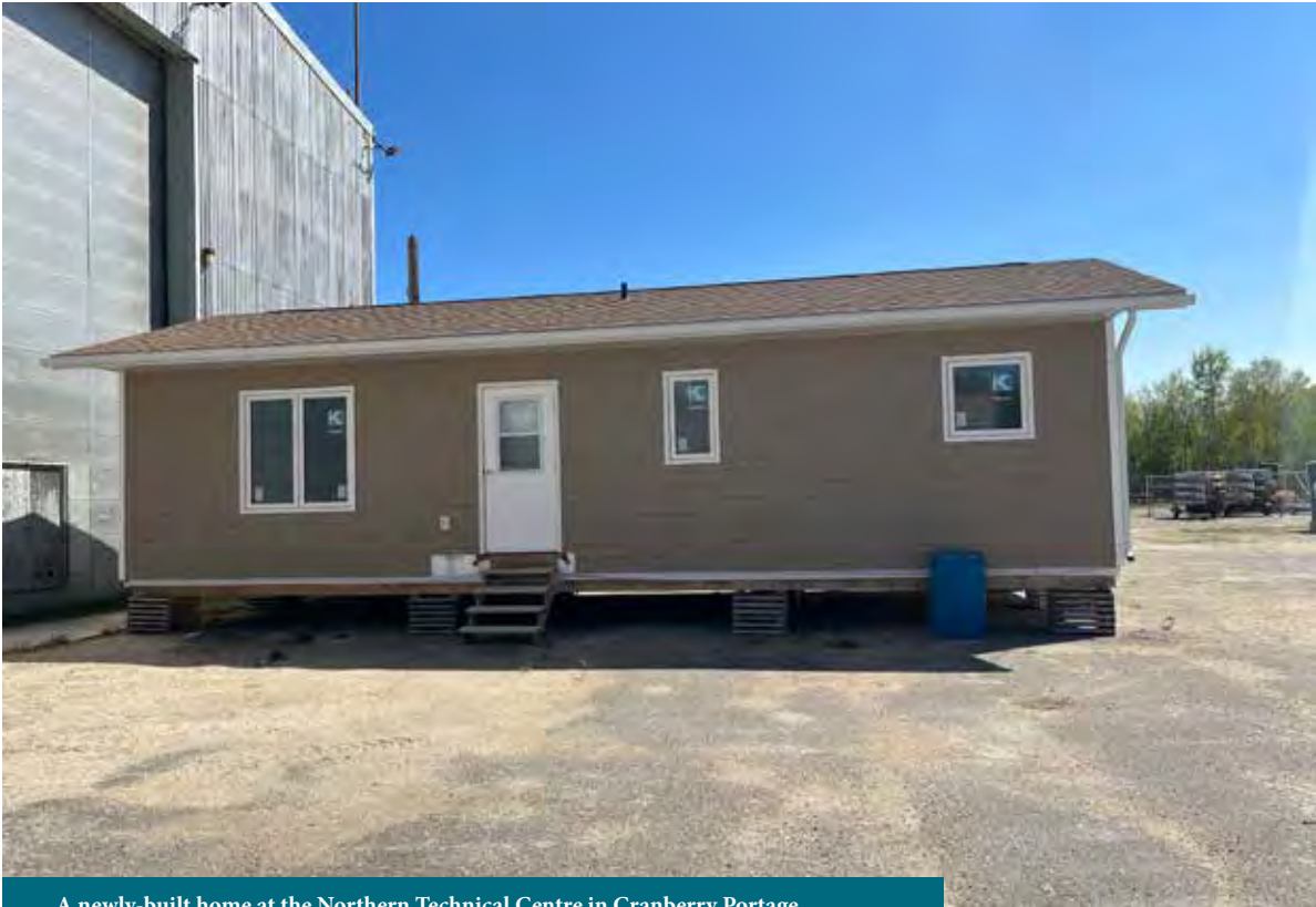
A newly-built home at the Northern Technical Centre in Cranberry Portage.
