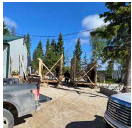
June 2024 4 + 1 Carpentry students building sheds.
